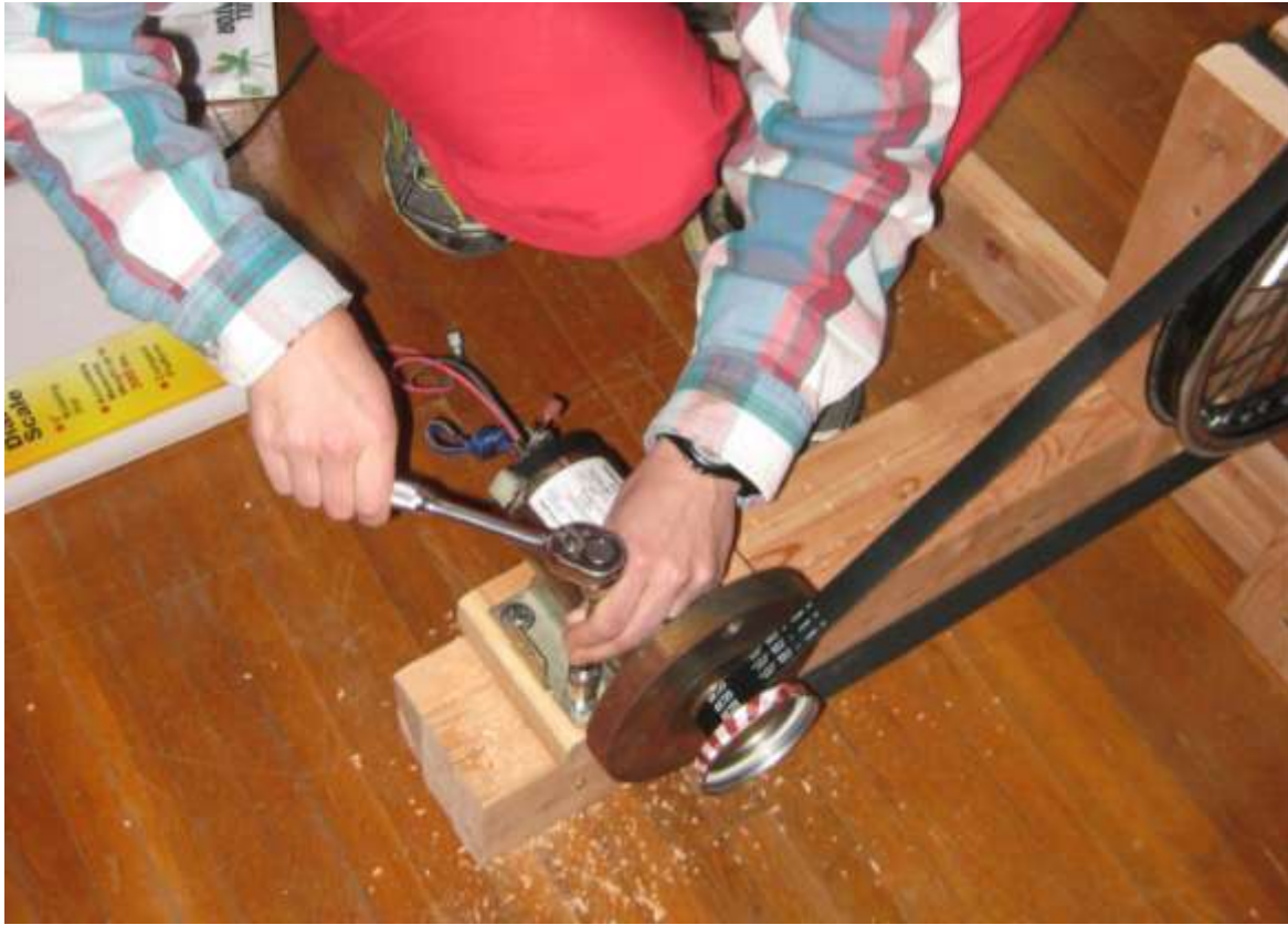
Figure 9: attaching the generator
